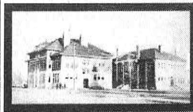
The old high school buildings were torn down and the new building built on the same site
