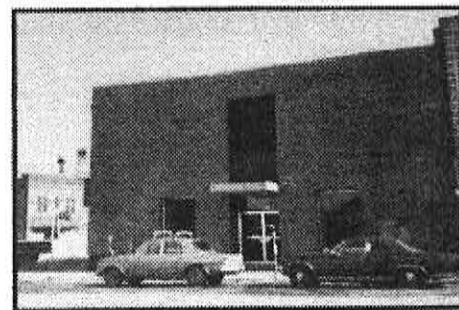
Building front after renovations done in 1966
