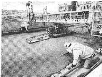
Crews smoothing concrete
